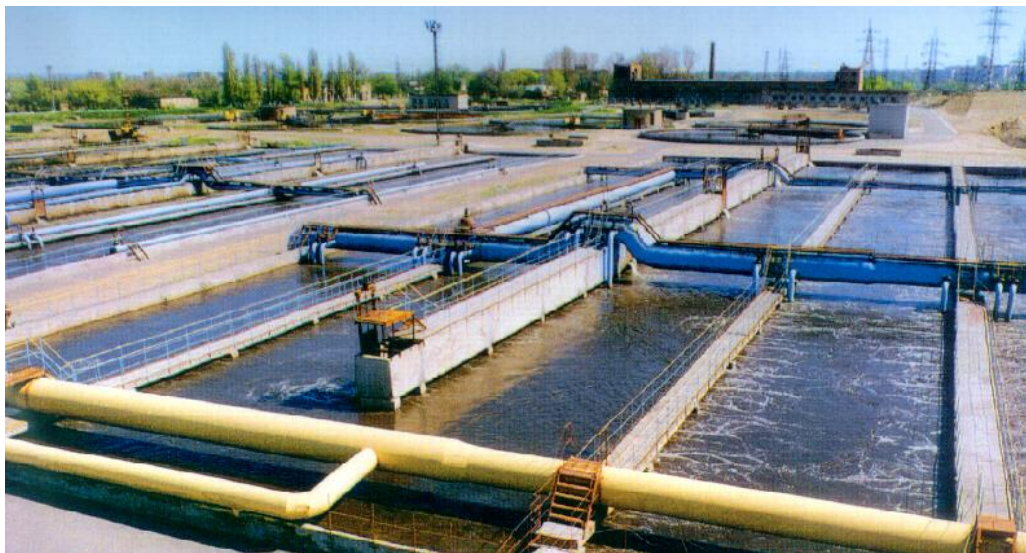
Fig. 2.32. General view of the aeration tank
